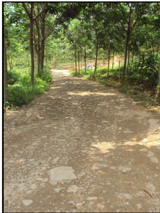
Photograph showing access road maintained by paving granite stone
